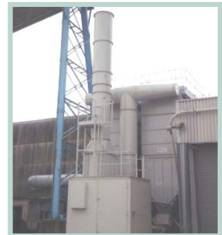
Cutting, trimming and finishing gypsum products
