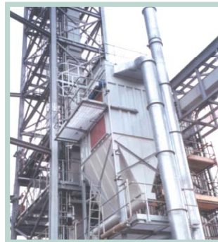
Dockside handling, conveying and storage, of grain
