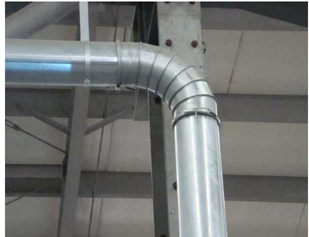
Put O-ring on cut duct, slide slip duct over cut piece of duct
